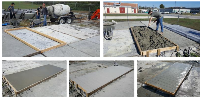
Figure 28: Electrical system concrete slab construction.
