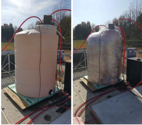
Figure 35: Filling and insulating the aboveground storage tank.
